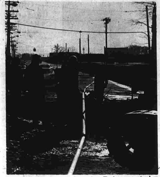
The emergency sewer bypass can be seen here. The bypass was rigged when the existing line broke after a cave-in. The metal line runs over the excavation and into a manhole below the work area. (Herald photo by Pinto)
